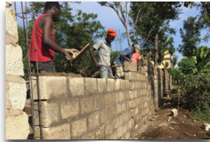
Completing the Security Wall
