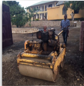
Paving the Parking Lot
